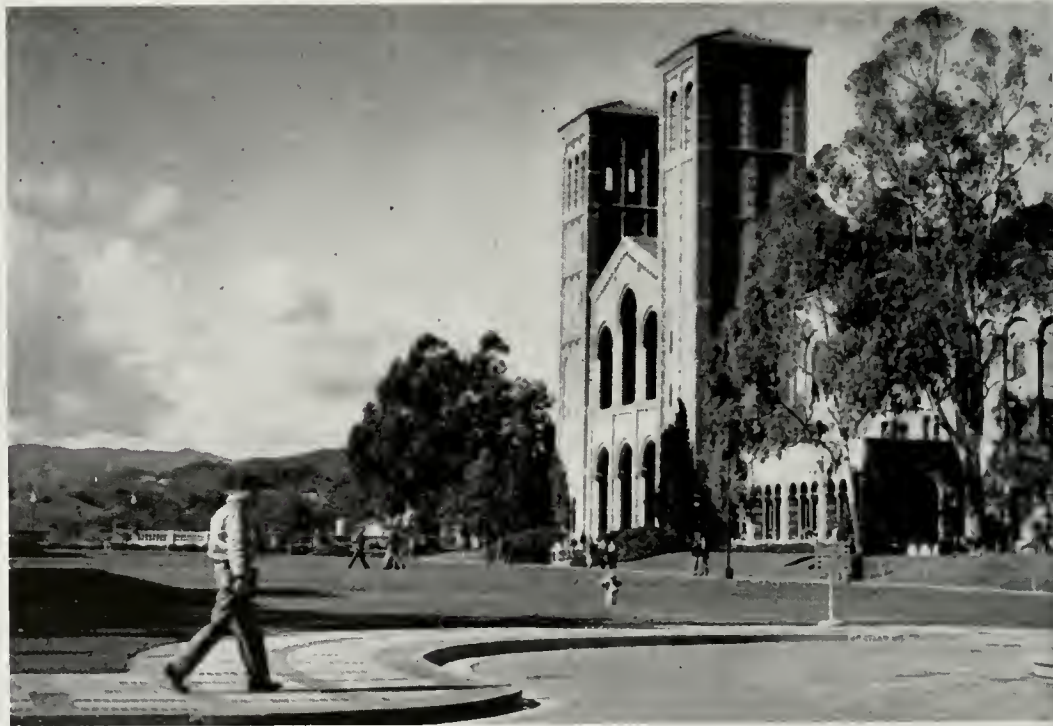
AT LOS ANGELES: acquisition of a chancellor and increased local administration was a welcome accompaniment to the forty-one million dollar construction program in progress on the UCLA campus. Newly-completed law and art buildings will be joined by others including a medical school.
